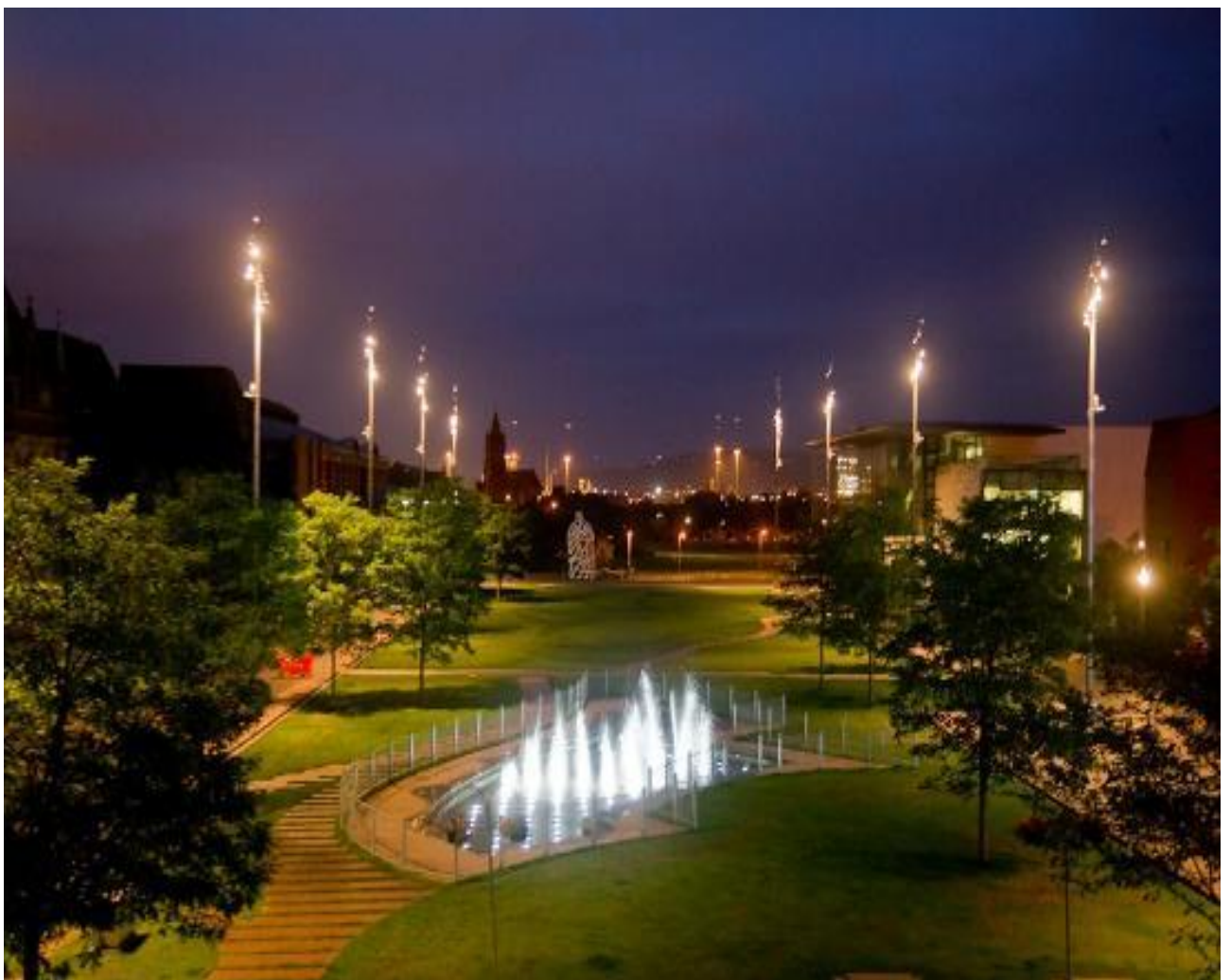
Middlesbrough Centre Square
